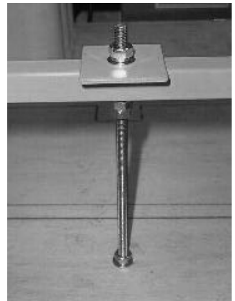
Closeup of battery holddown bolt/plate
